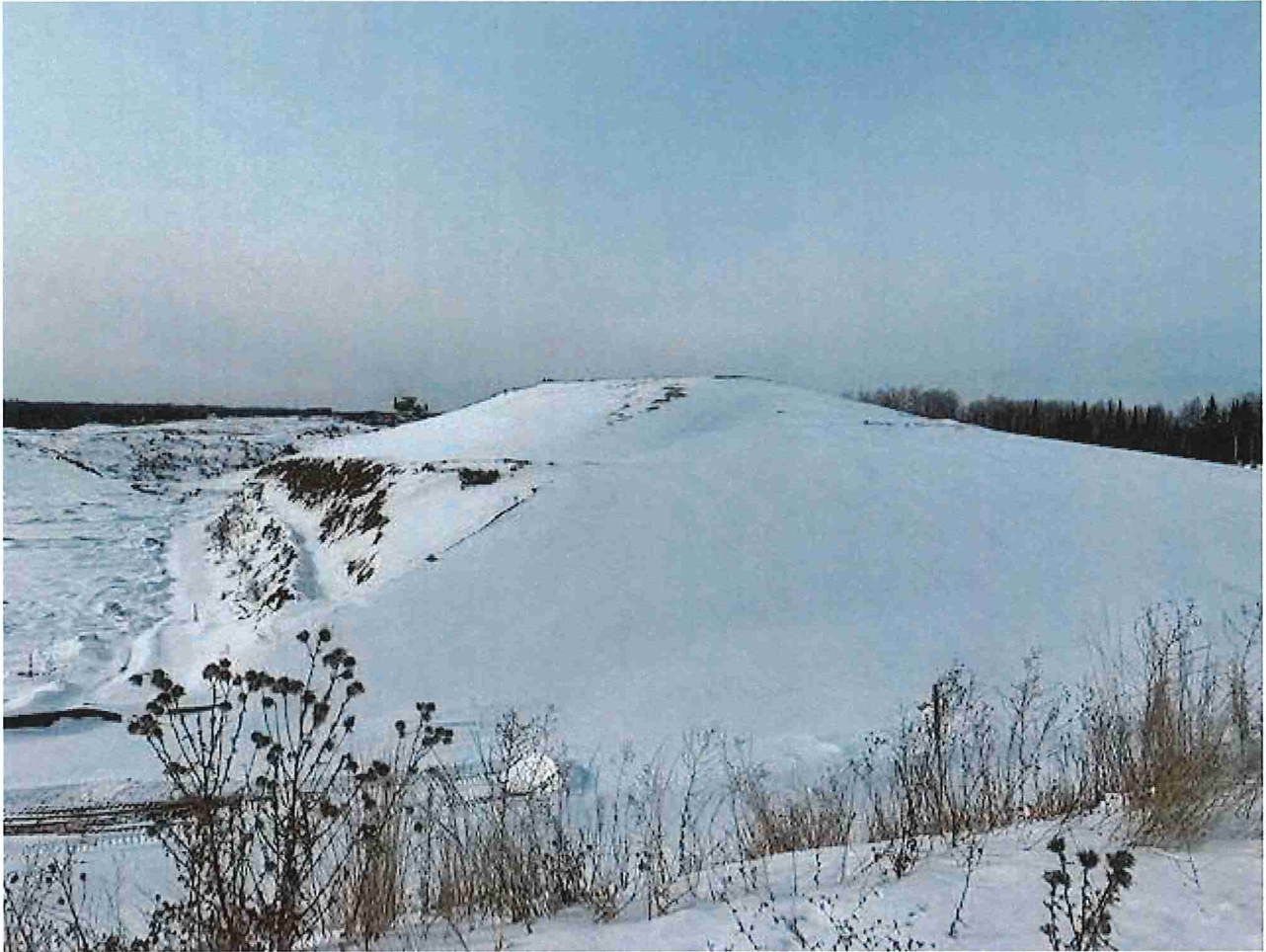
Photo 1 – Eastern and southern slopes of industrial cell B-1 as viewed from southeast corner, facing northwest.
